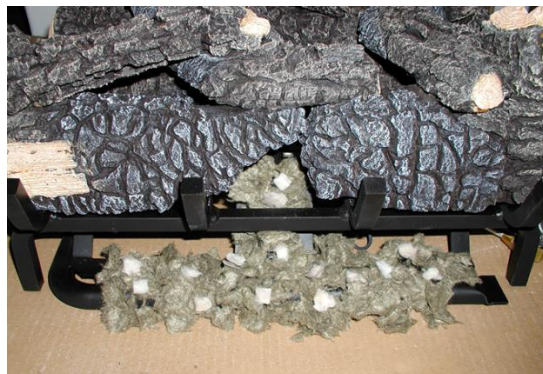
Front Burner with Embers Properly Installed
